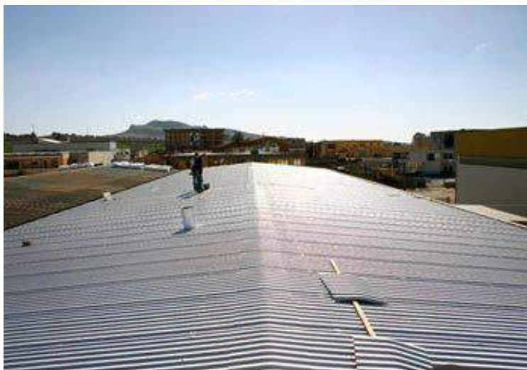
Figura 32: POST-OPERAM (COPERTURA IN PANNELLI SANDWICH)
